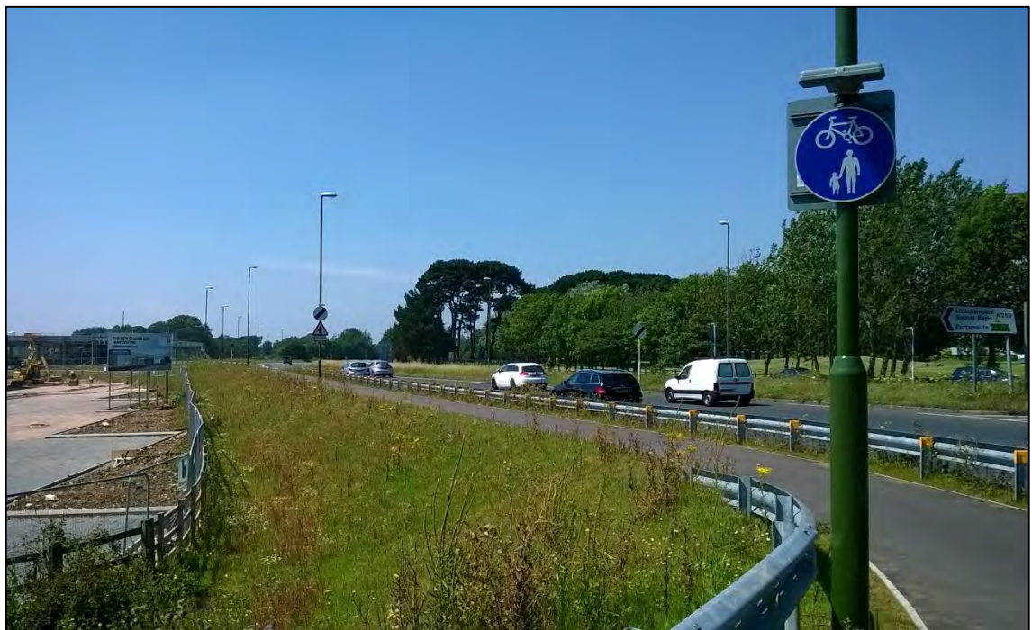
Figure 3.1: Shared Footway/Cycleway adjacent the A259 New Road
