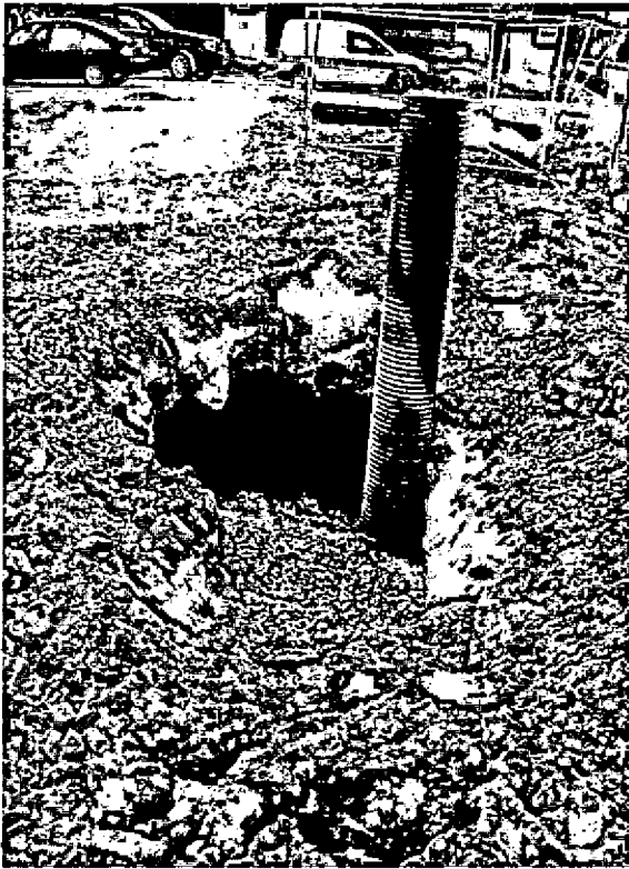
Figure 33: 26 March 2008 – extraction sump pipe
