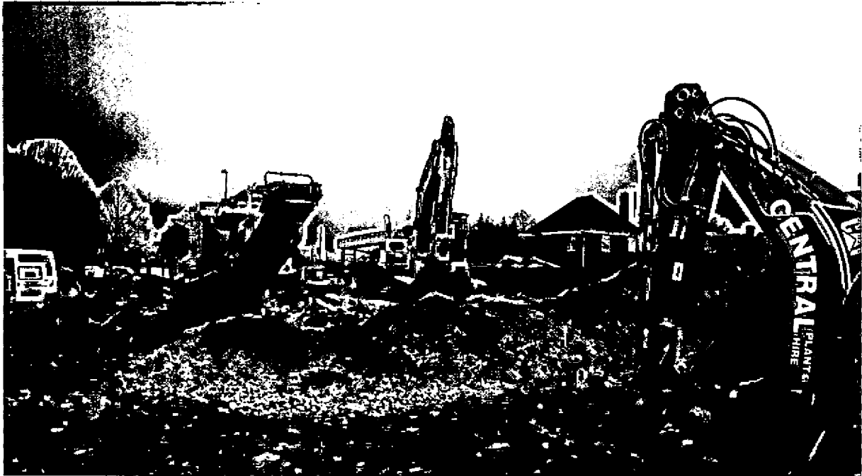
Figure 26: 7 February 2008 -General view towards north-east corner showing stockpiled crushed concrete.
