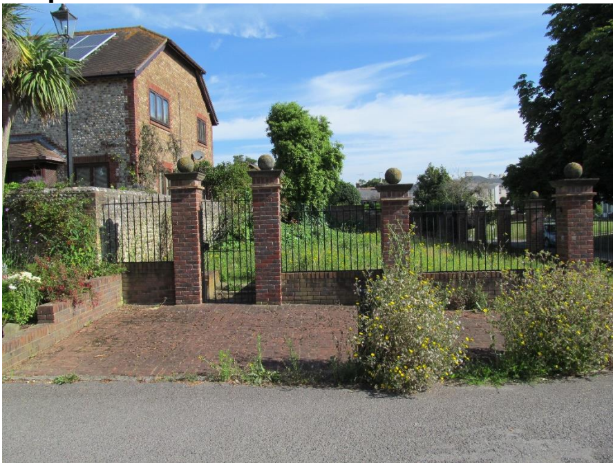
Existing Pedestrian gate, Wall, Pier, Railing and hardstanding between road
