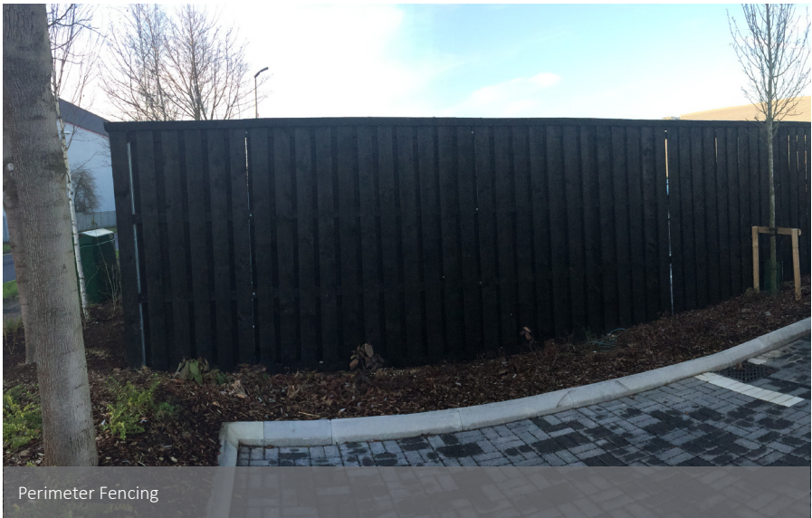
Stained timber boundary fence (Ref:3068-60A)
