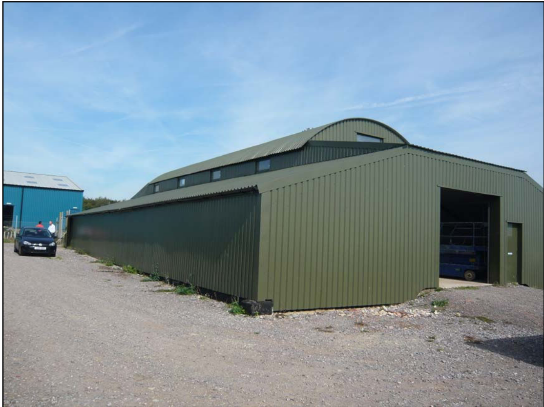
Fig 1 Yarmer Barn from the south west
