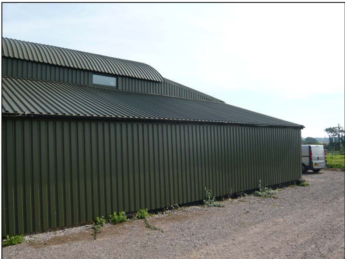
Fig 2 The western elevation of Yarmer Barn
