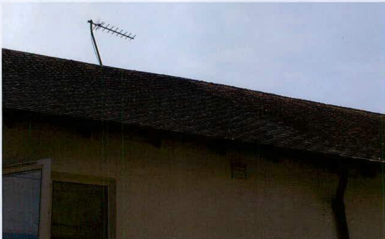
Photograph No. 17 - Roof tiles are tight-fitting with no visible opportunities for bat roosting. The photograph is typical of the general state of the main residential property on site with ' negligible ' bat roost potential.
