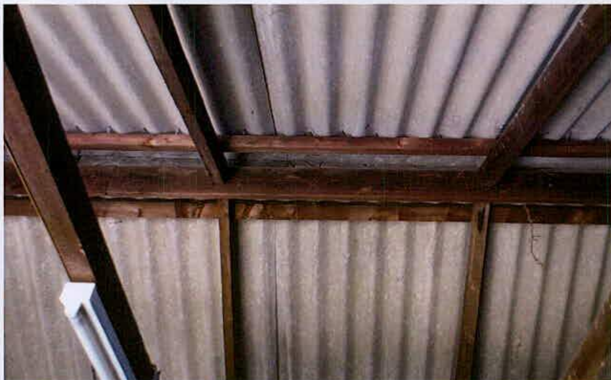
Photograph No. 19 - Roof section of the subsidiary out-building on site with ' negligible ' bat roost potential.
