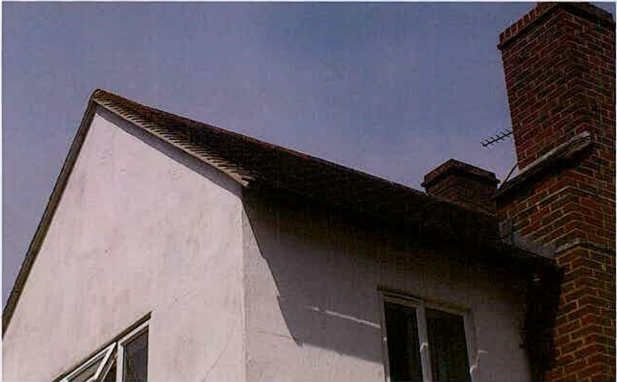
Photograph No. 15 - Mortared edges of the existing property roofline are intact. The photograph is typical of the general state of the main residential dwelling on site with ' negligible ' bat roost potential.
