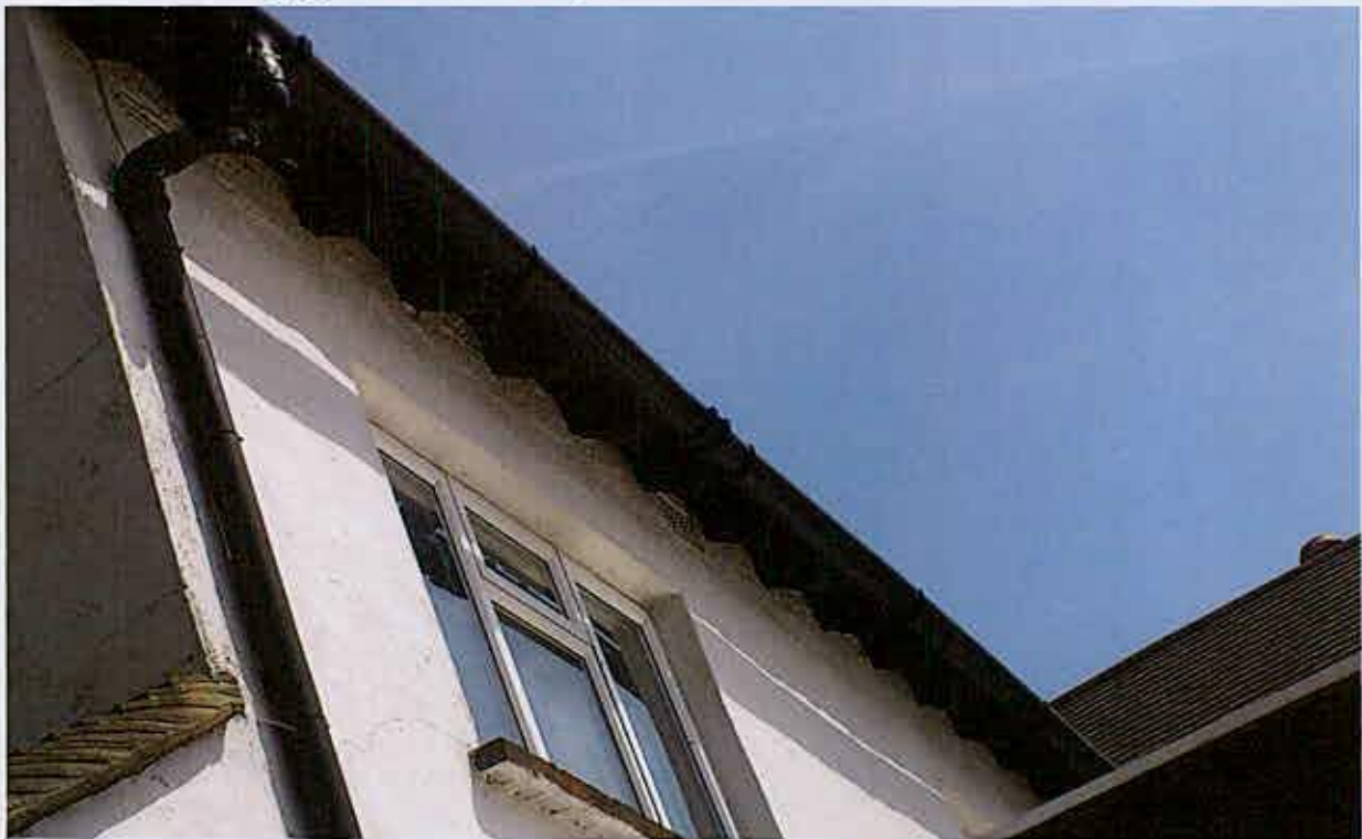
Photograph No. 16 - Eaves of the property roof are intact. The photograph is typical of the general state of the main residential dwelling on site with ' negligible ' bat roost potential.
