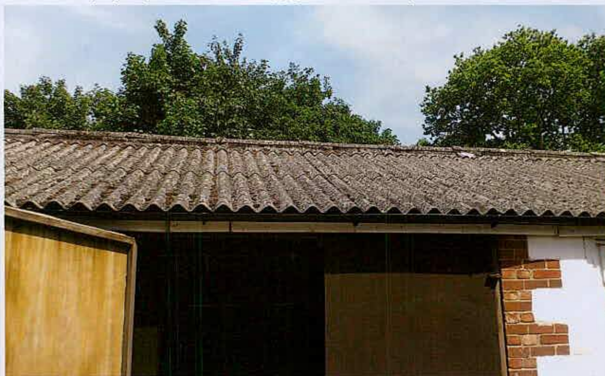
Photograph No. 18 - Subsidiary out-building on site - asbestos roof with no lining and very little opportunity for bat roosting with ' negligible ' bat roost opportunity and potential.
