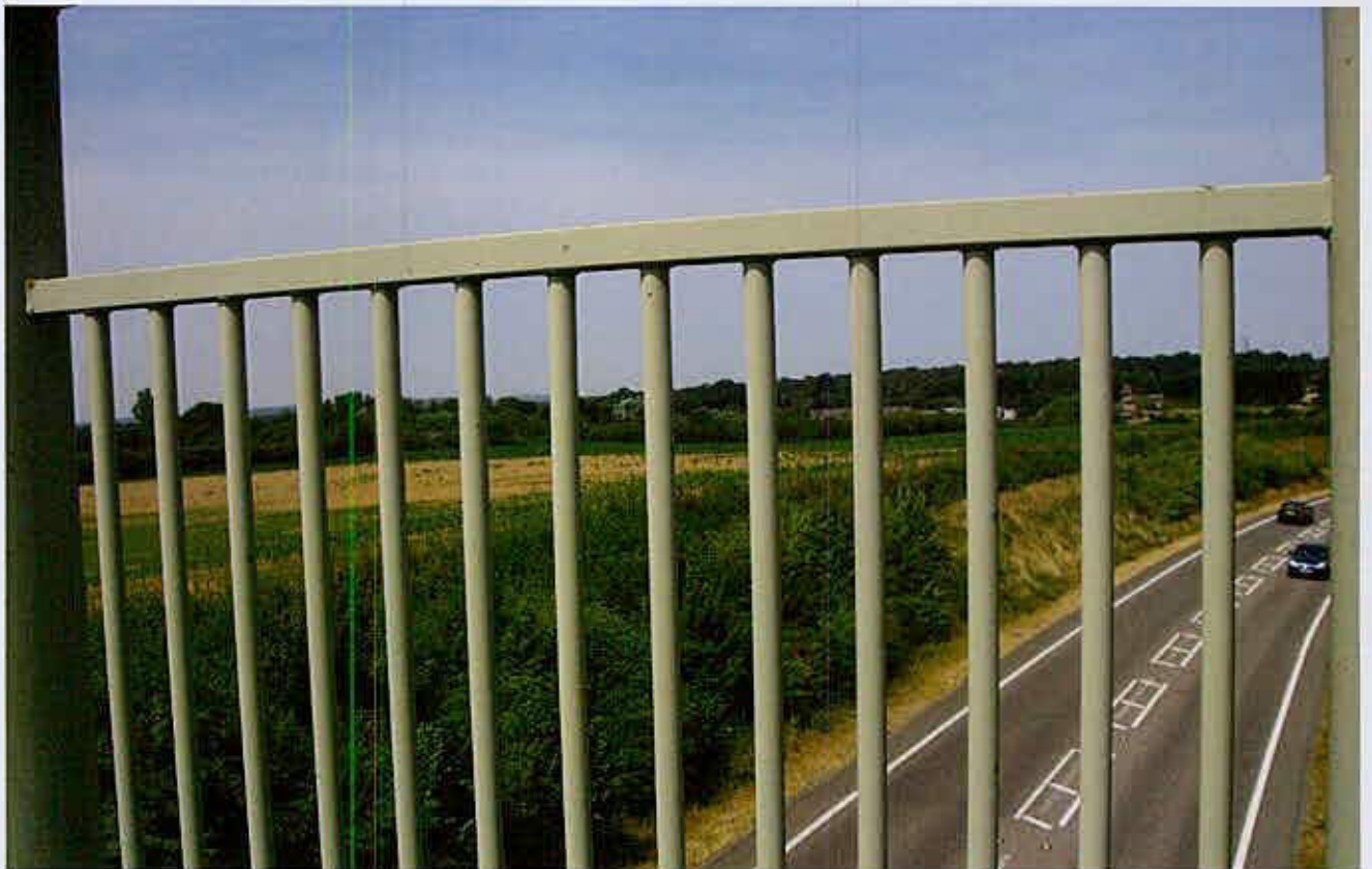
Viewpoint No 10: A280 Footbridge; Public Right of Way (3692); View north west
