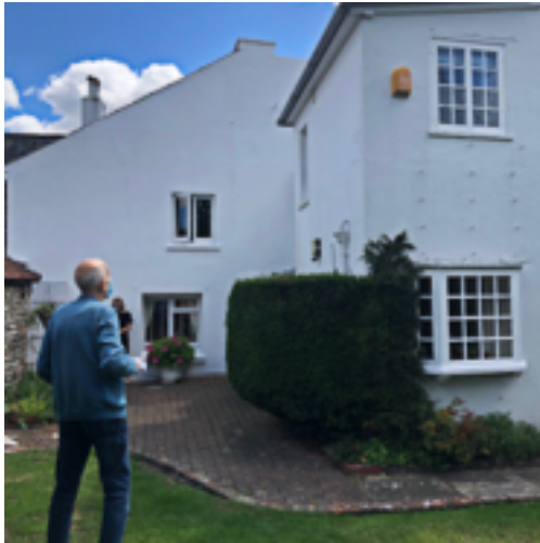
Back elevation - east. Note: kitchen window, room 11, lhs + bathroom window, room 23, above
