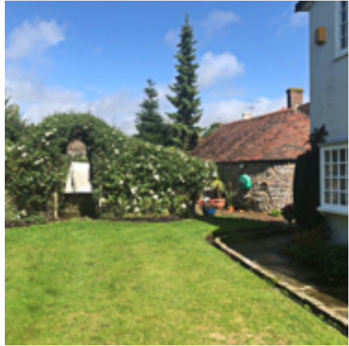
Gardens, back elevation + outbuilding - west
