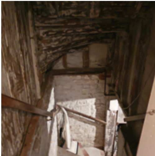
Staircase, ground floor to basement
