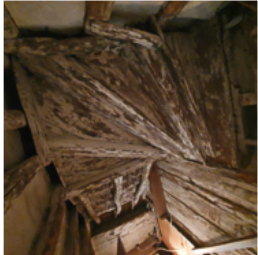
Staircase, ground floor to basement
