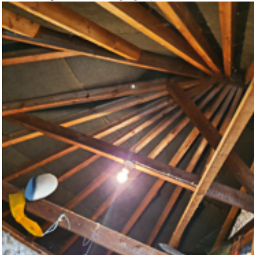
Roof structure, outbuilding
