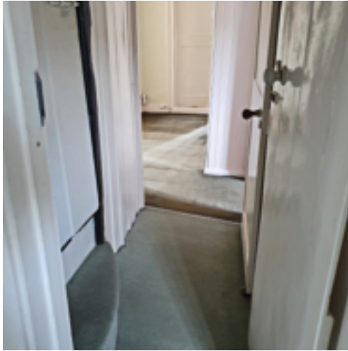
Corridor (20) leading to bathroom (23)
