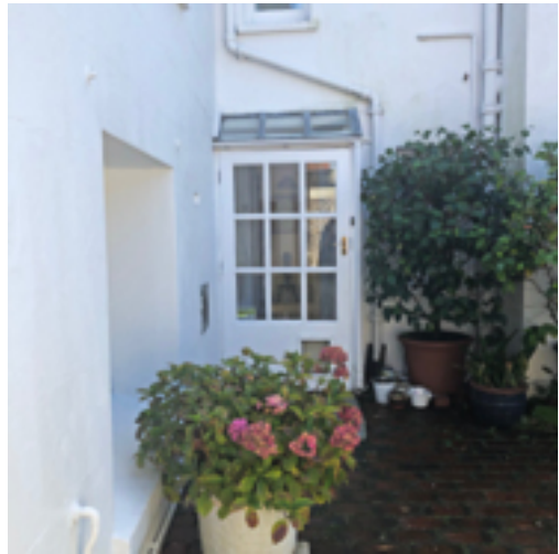
Back elevation, porch, room 7
