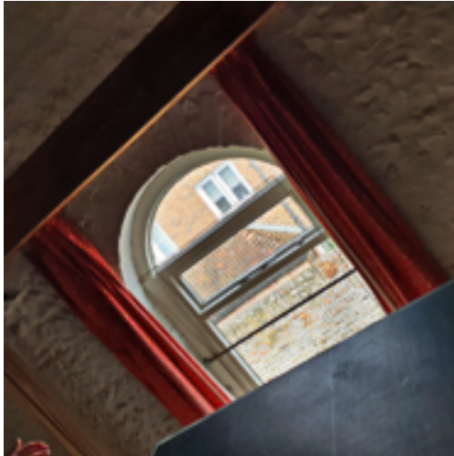
Hayloft (22) window, north elevation
