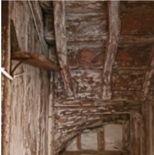
Staircase, ground floor to basement
