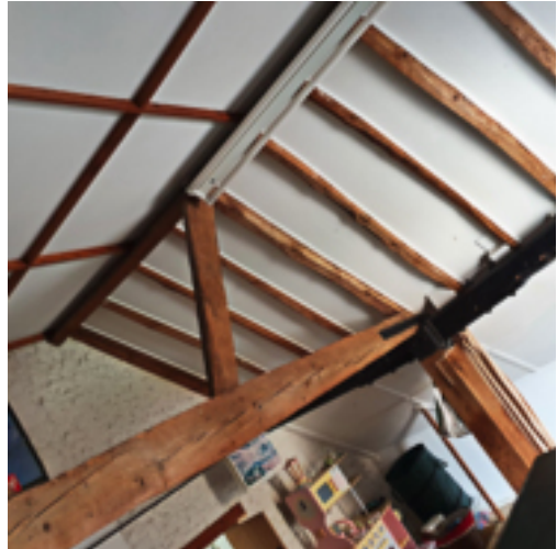
Hay loft (22) - ceiling structure
