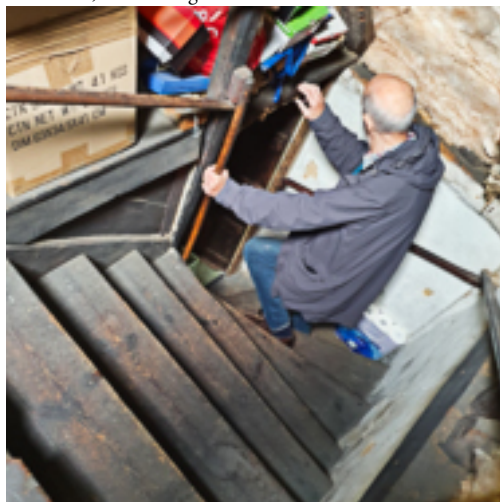
Staircase - 1st floor to attic
