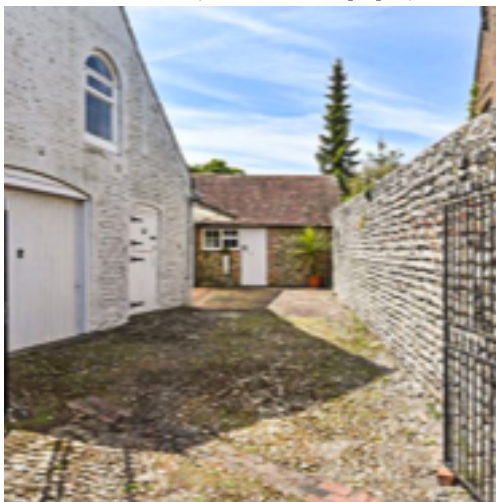
Side elevation, stables, north; outbuilding, at back of photo.
