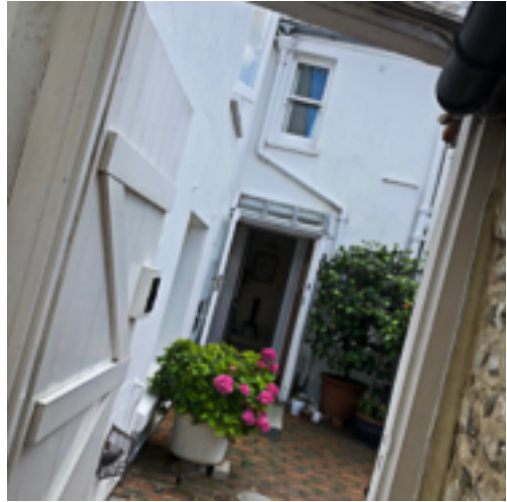
Back elevation, porch, added circa 80's room 7
