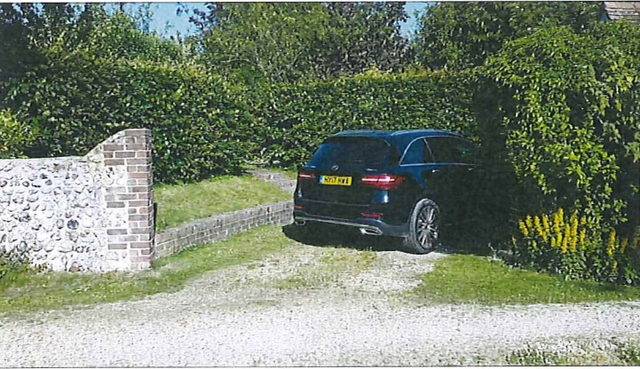
PICTURE OF EXISTING WALL/PIERS
