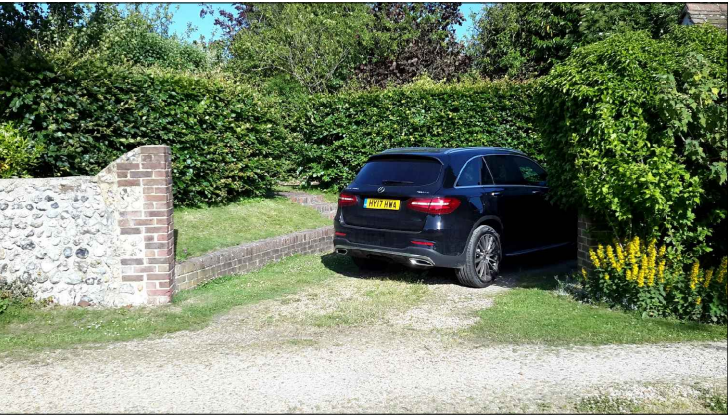
PICTURE OF EXISTING WALL/PIERS
