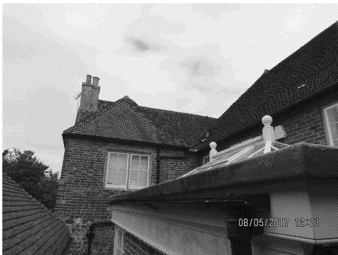
EAST ELEVATION OF REAR WING
