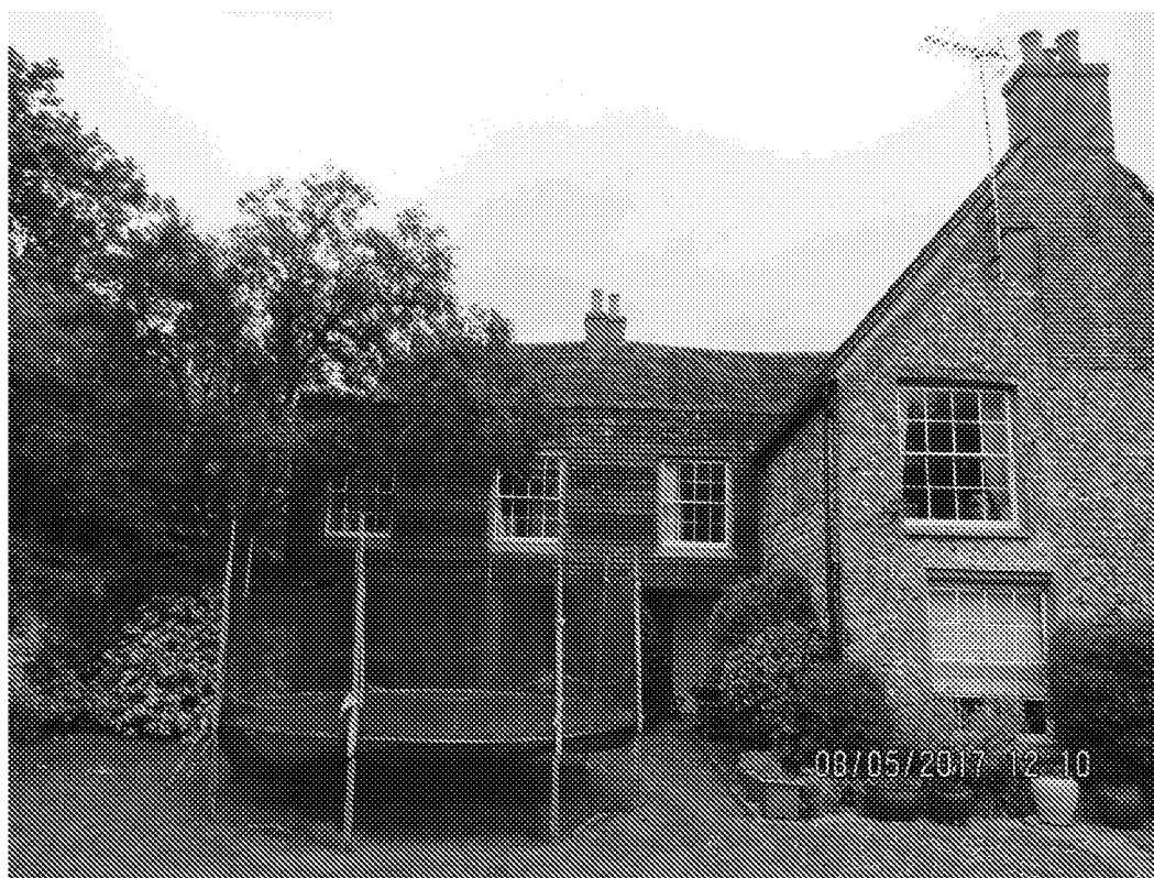
SOUTH SIDE OF MAIN HOUSE
