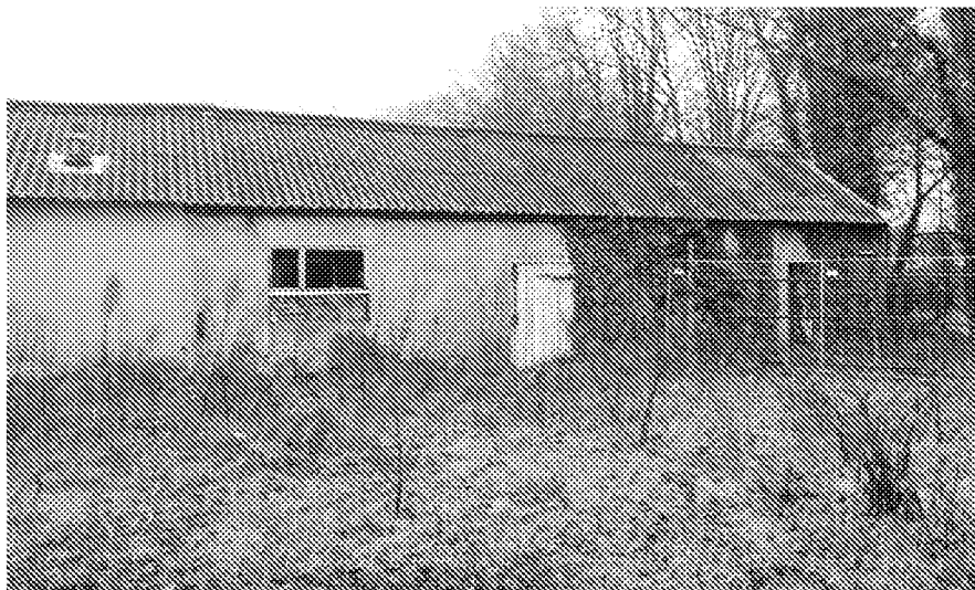
Photo 48 – Block E – View of side elevation
