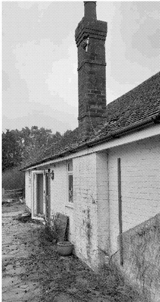
Photo 4 - Block A – Rear elevation showing chimney
