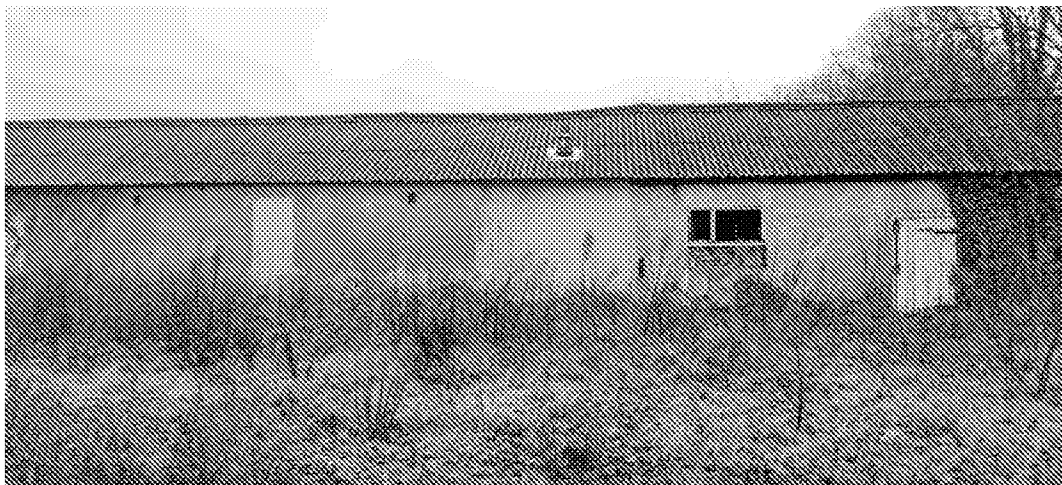
Photo 49 – Block E – View of side elevation
