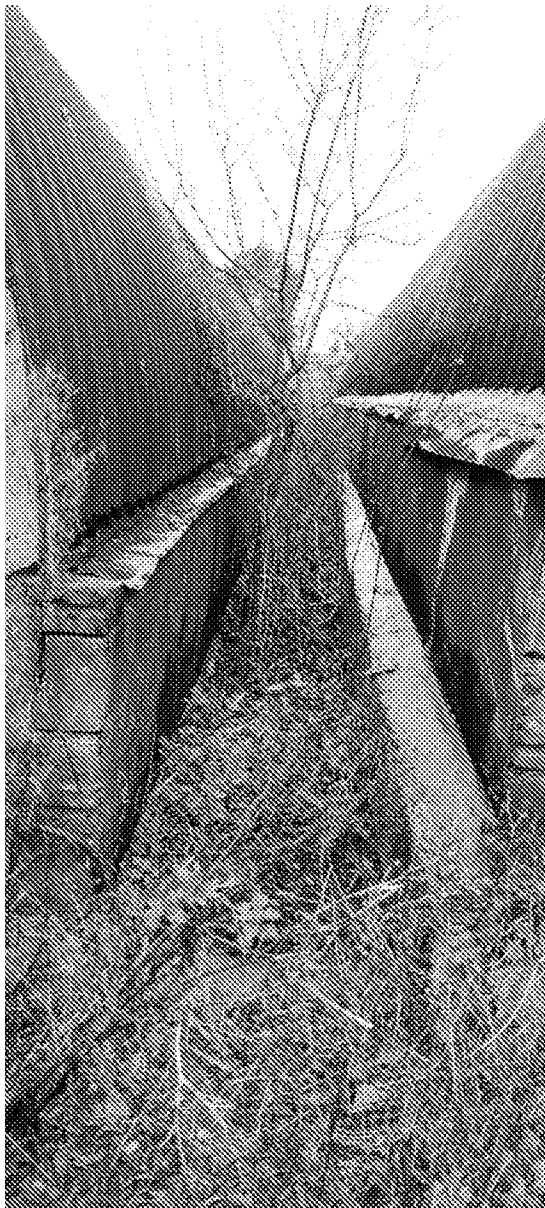
Photo 39 – Block C – View between two huts
