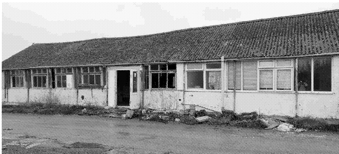
Photo 41 – Block D – Side elevation view
