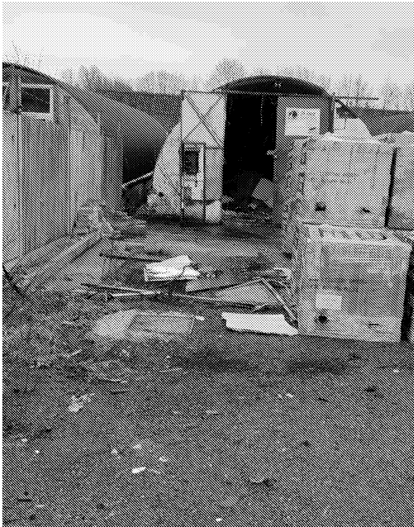
Photo 31 – Block C – Gable end of Hut C4
