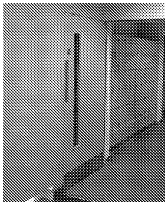
Where doors must swing out into a corridor they should be set in a recess
