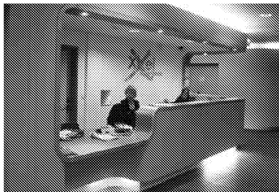
The reception desk is designed for use from both sides by people using wheelchairs
