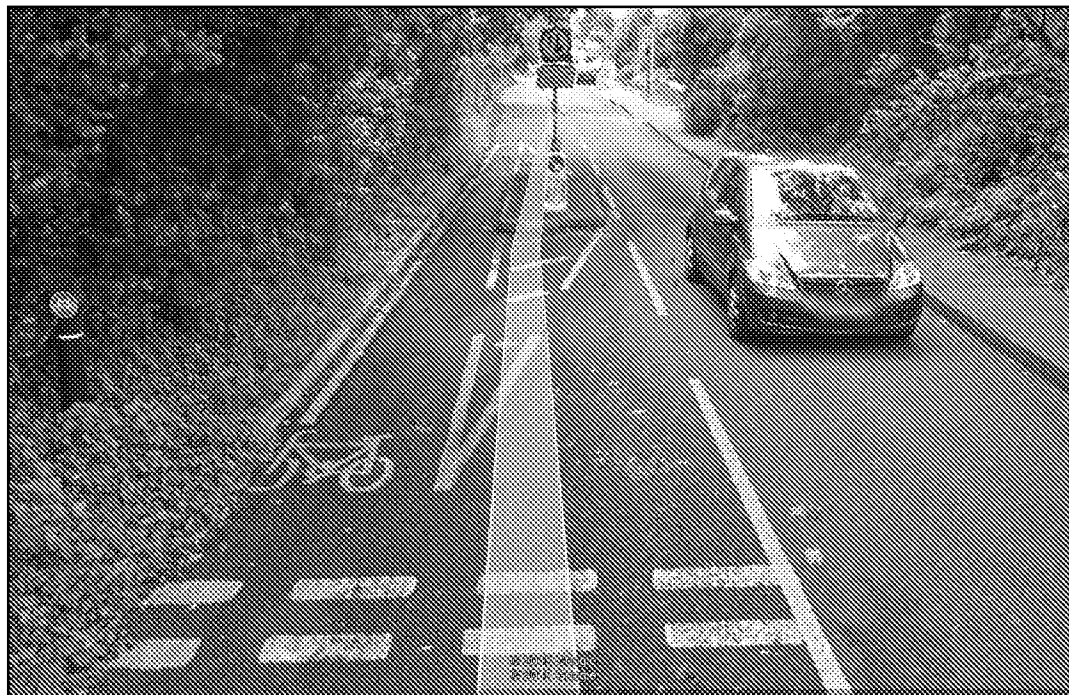
Figure 5.2 – Existing One-Way Priority System on Arundel Road
