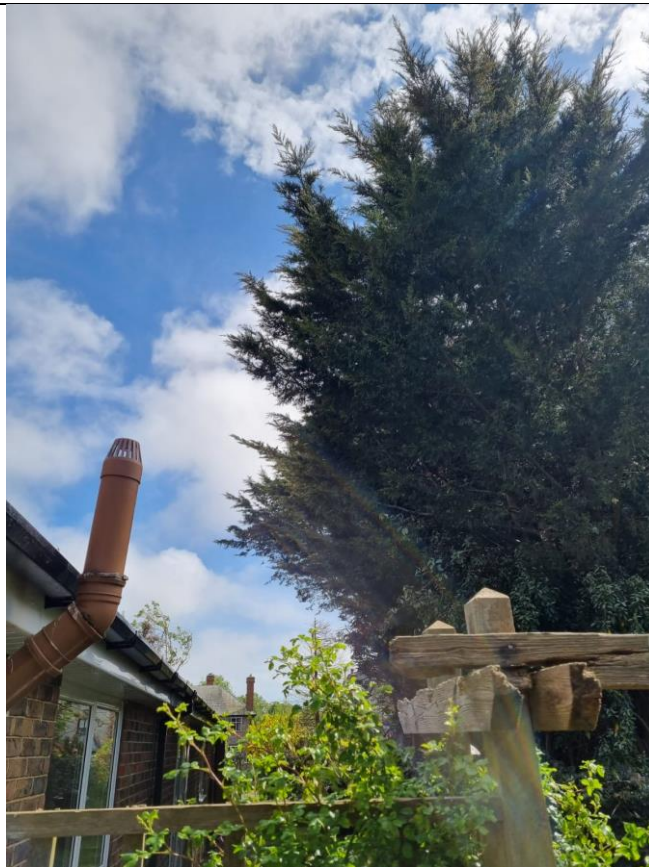
Picture 4 TG2 showing overhang and encroachment of living space
