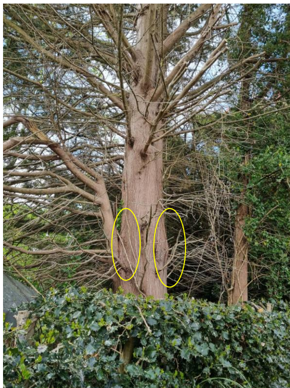
Picture 3. T1 from south east showing swelling at area of tight included bark union
