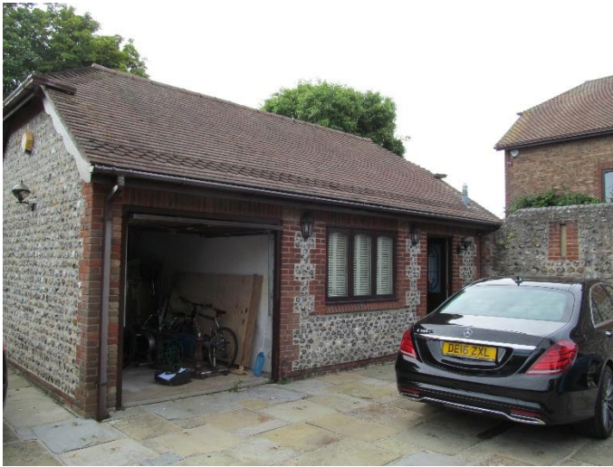
Front View Existing Garage
