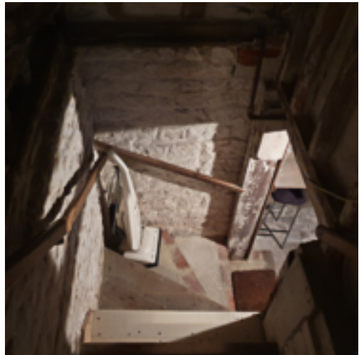
Staircase, ground floor to basement
