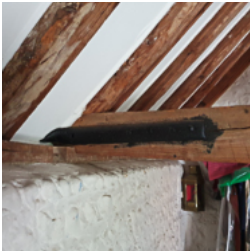
Hay loft (22) - rafter / wall junction
