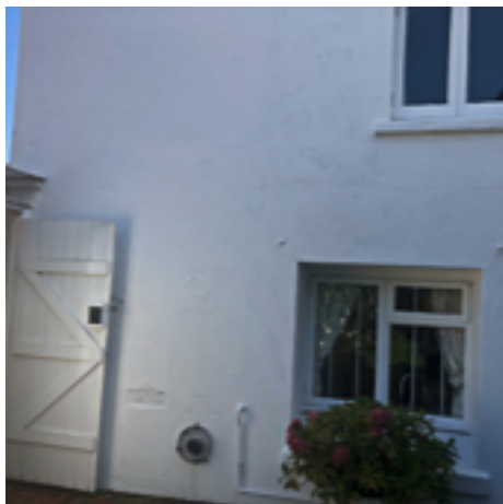
Back elevation, kitchen, room 11. Note: casement window, to be changed ref W2
