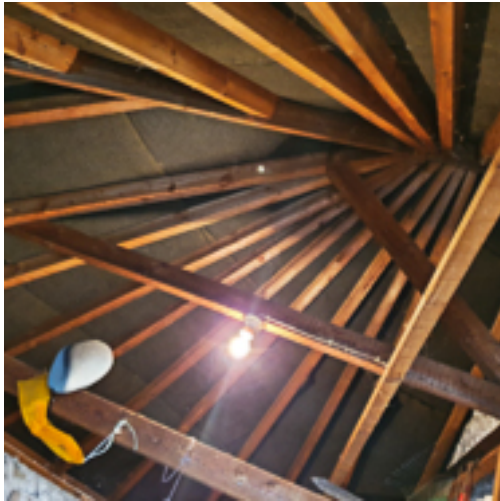
Roof structure, outbuilding
