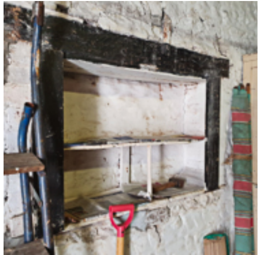
Alcove detail, outbuilding
