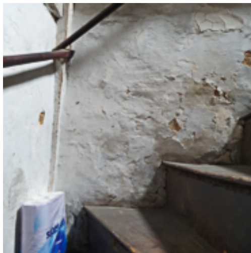
Side of stairwell wall to attic from 1st floor
