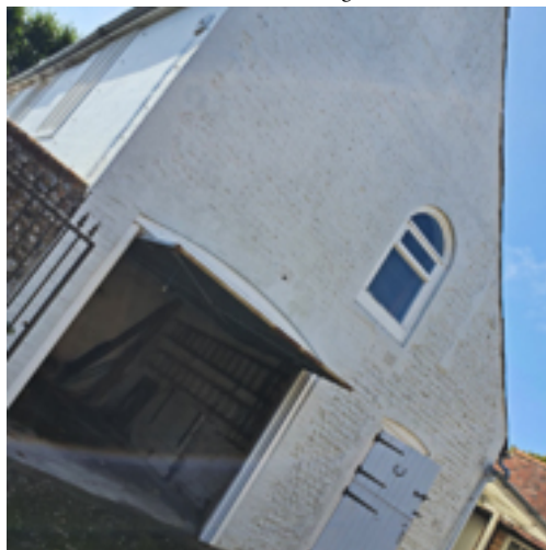
Side elevation, north - garage, (15), (old stables) and store. Note: stable door, retained but to be fixed shut (14)
