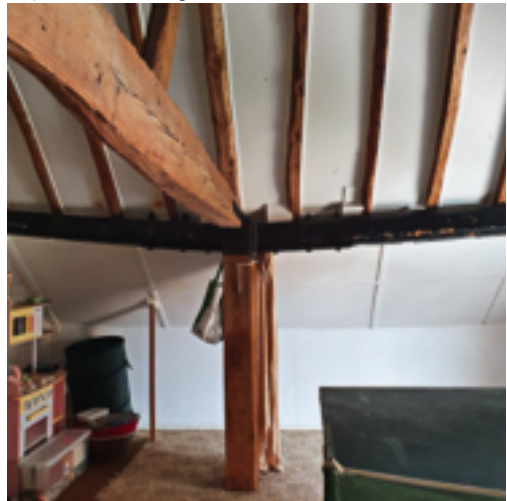
Hay loft (22) purlin, tie beam and post
