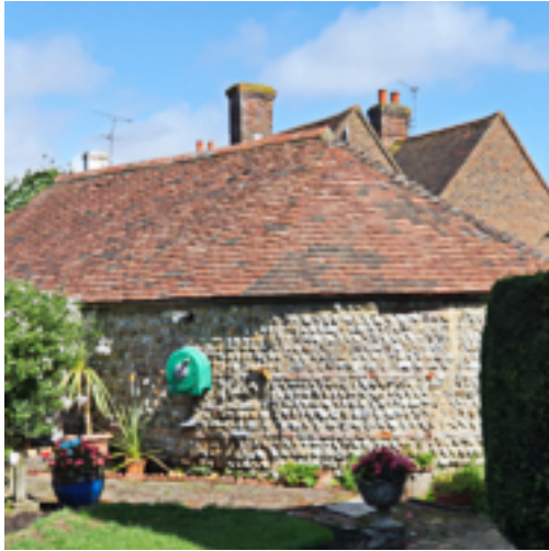
Outbuilding - north end of property
