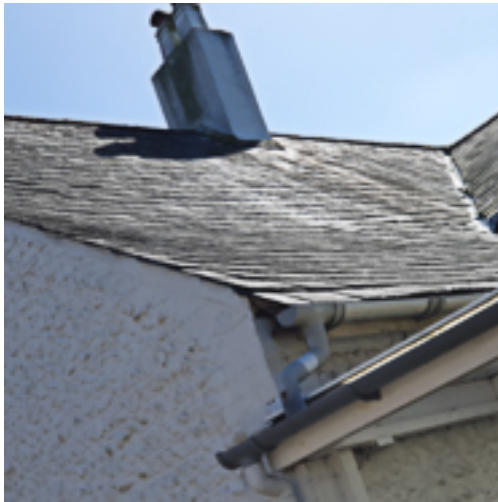
Roof over old stables/hayloft, room 22
