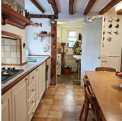
Kitchen (11) looking toward utility (12) - proposed changes - remove infill between beam and post structure, retain structure
