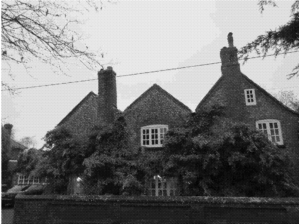
▲ 3 South facing gable wall (westernmost chimney stack shown to the left)
