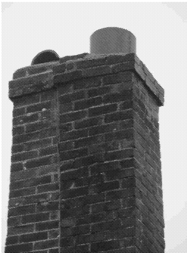
▲ 8 Westernmost stack constructed at later date to follow 'lean' of eastern stack
