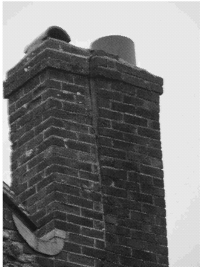
▲ 4 Stack comprises 2no separate flues 'butted' together – straight vertical joint
