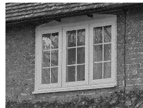
Casement windows with glazing bars
