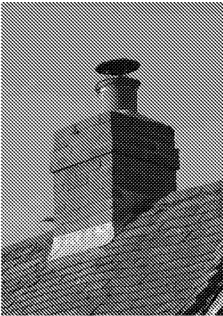
Chimneys on key plots
