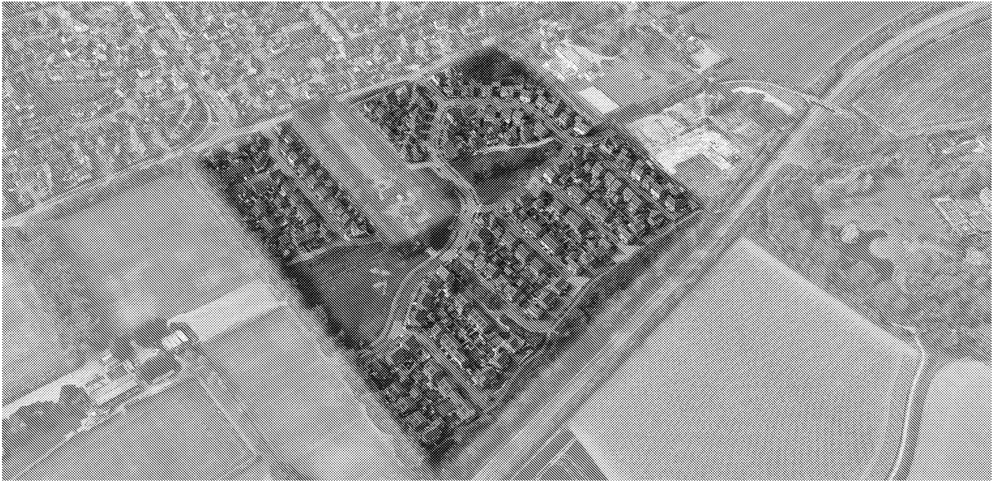
Aerial view (Google Earth)
