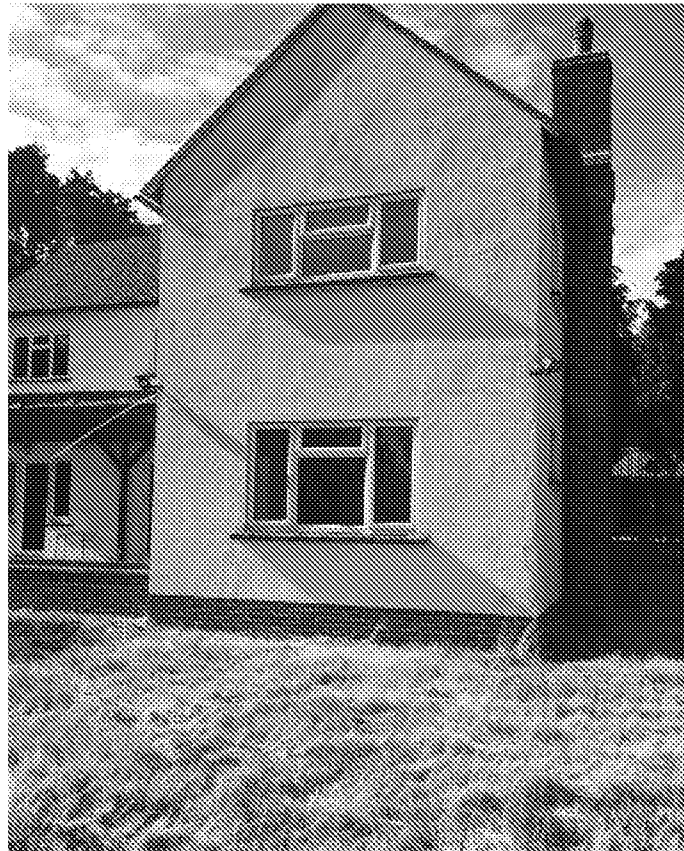
The dwelling - southern elevation
