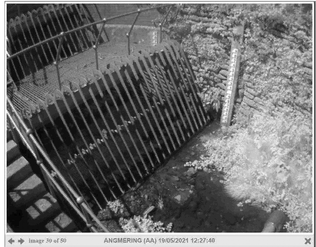
Figure 4. Webcam image, Black Ditch culvert entrance, Water Lane
