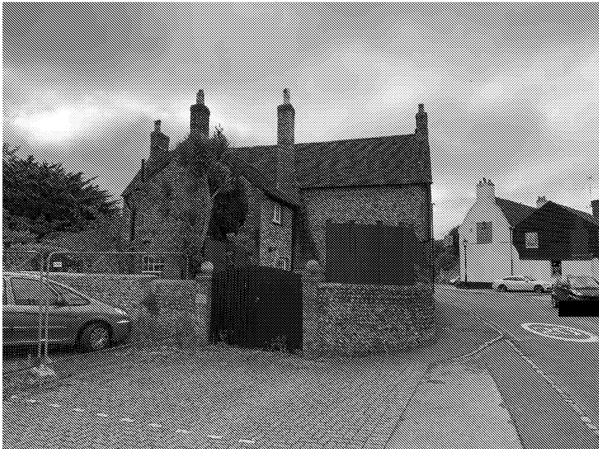
Figure 15: Eachways to the left, with the gable end of The Lamb Inn to the right, from the garage site entrance on Water Lane.
