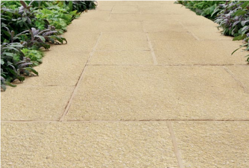
Paving slabs in buff finish to patios and communal terrace
