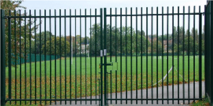
Automated double leaf swing gates with vertical bar square railings
