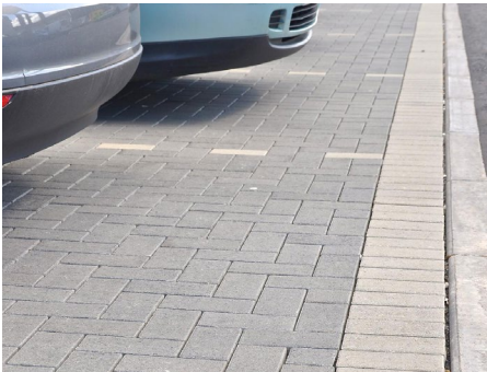
Permeable block paving parking bays
