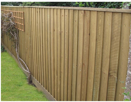
Closeboard fence to screen air source pump
