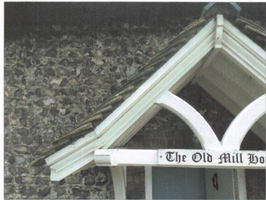
FRONT PORCH ROOF
