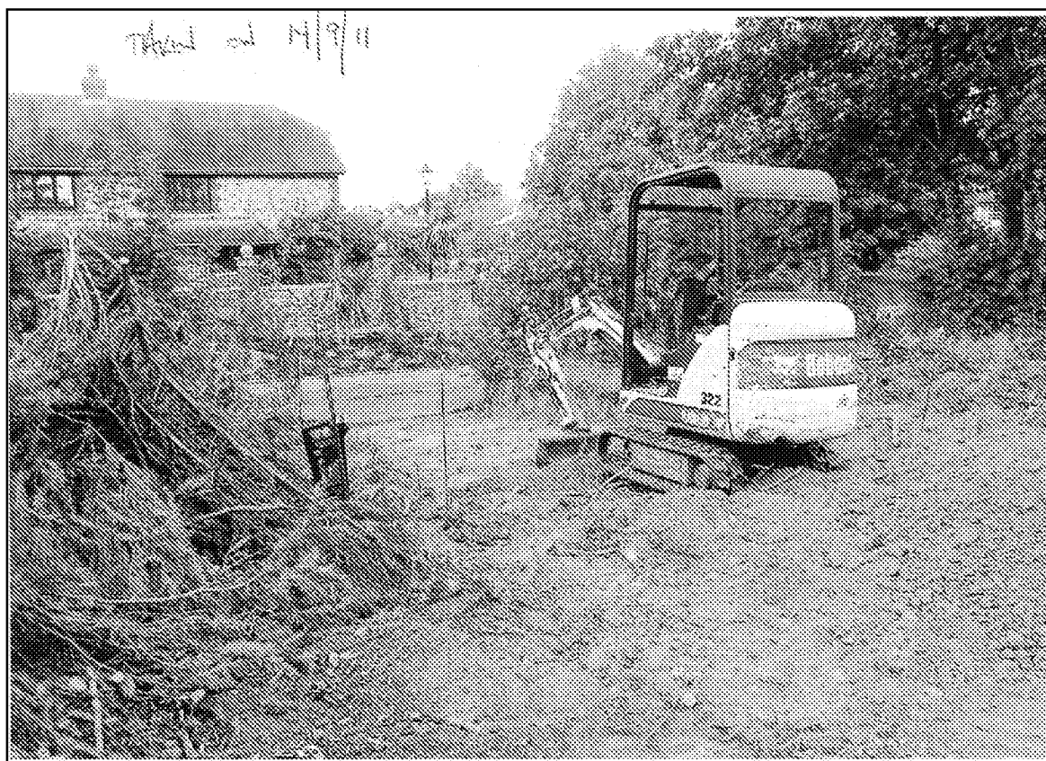
PHOTOS TAKEN 14/09/2011 ILLUSTRATING COMMENCEMENT OF ACCESS WORKS
