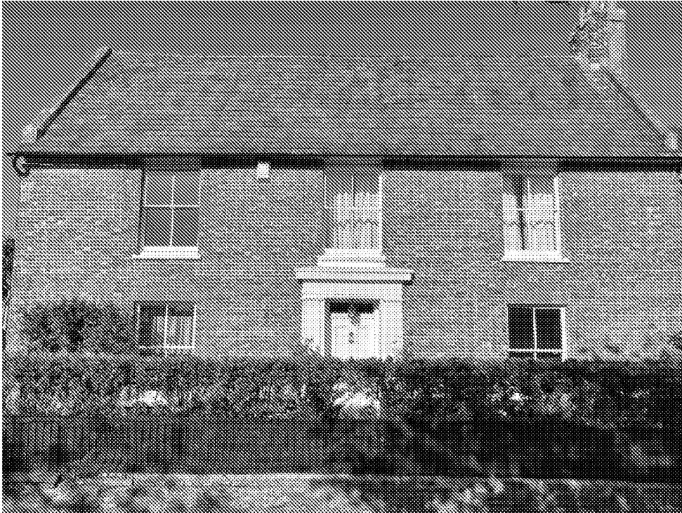
Five replacement sliding sash windows on Front elevation
