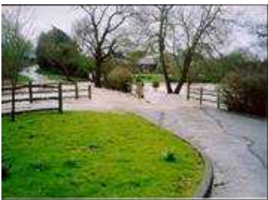
Avenals Farm pond overflows as the flow exceeds the capacity of the culvert under the access road
