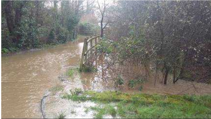
Culvert under A280 by-pass at junction with Ecclesden Lane
