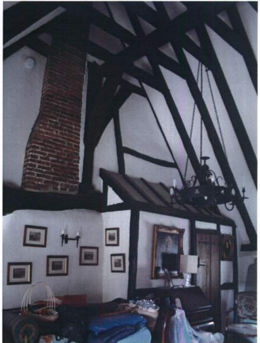
Fig.5: Crown Post roof structure now evident in core of house
