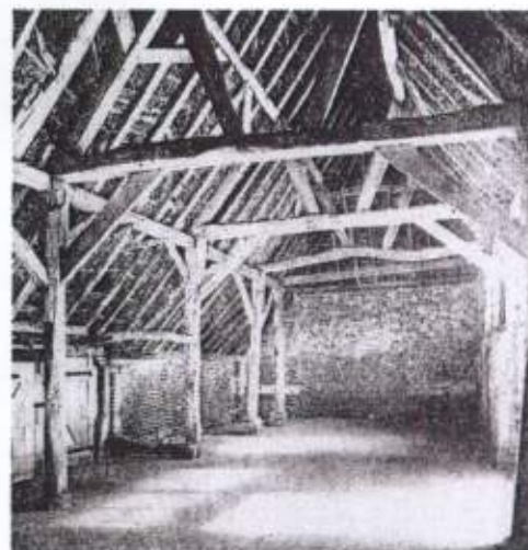
Fig. 15: Interior of Barn 1937, showing light from large windows still extant on South side.
