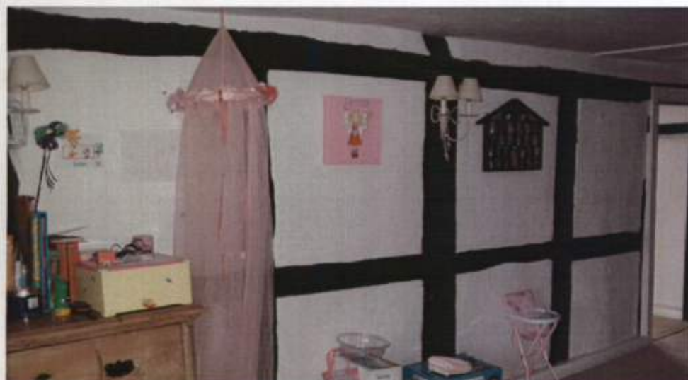
Fig. 7: Former external wall at first floor
