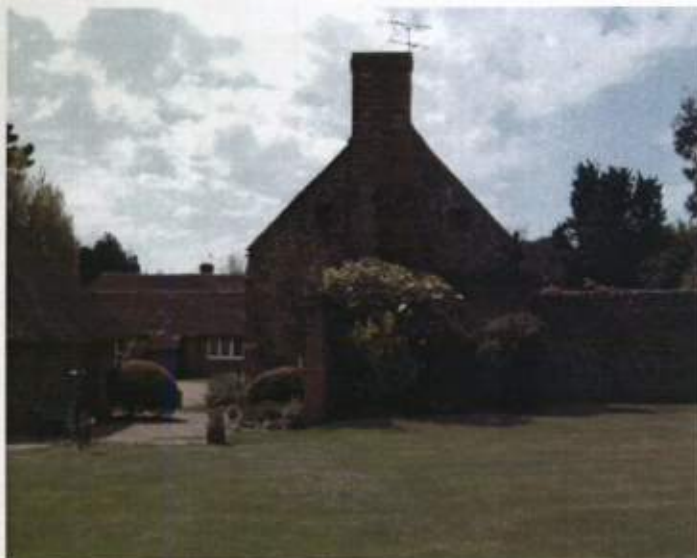
Fig.34: View of North elevation of Pigeon House showing flint wall to be retained in foreground.
