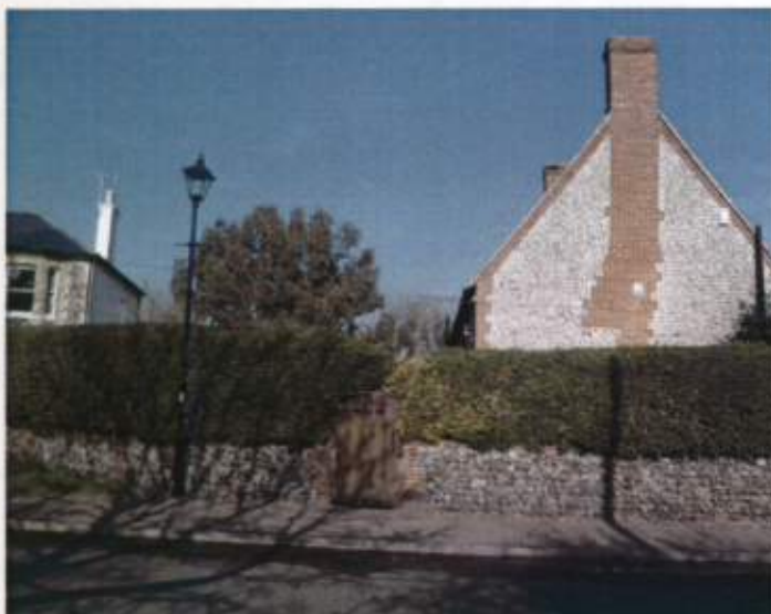
Fig.36: View of South elevation of Pigeon House from High Street
