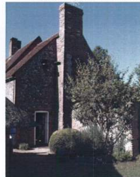
Fig. 9: Pigeon House from the North showing different ridge heights
