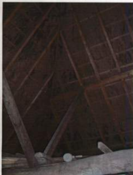
Fig. 17: Modern roof structure to Workshop
