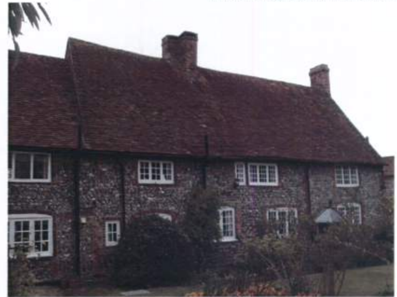
Fig. 13: Rear (West) Elevation; note straight joint to r/h side
