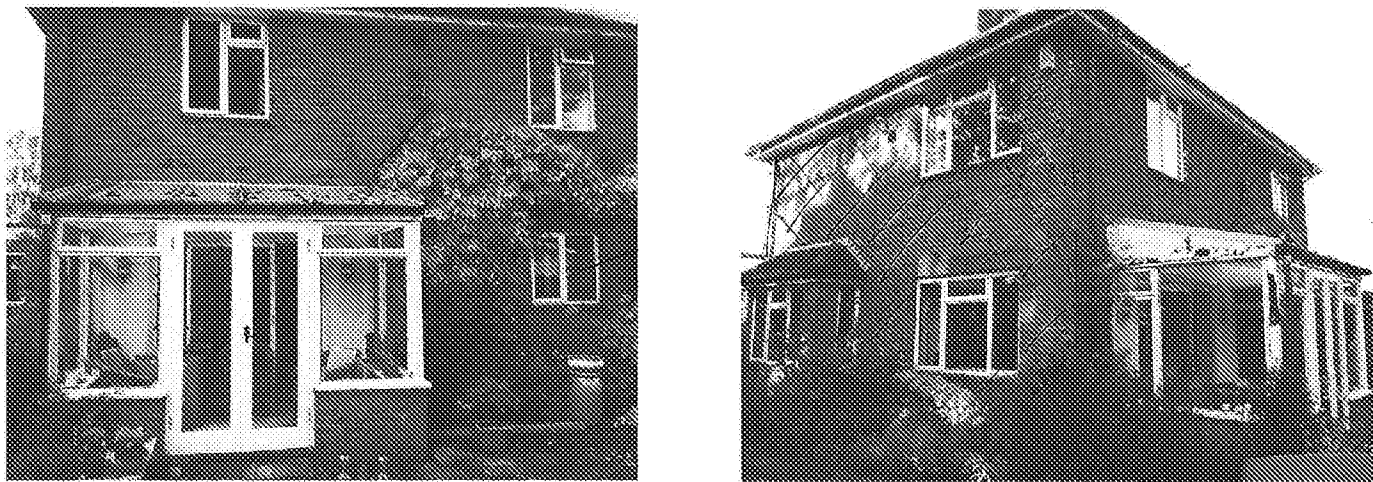
Photos showing rear and side house elevations and the existing conservatory
