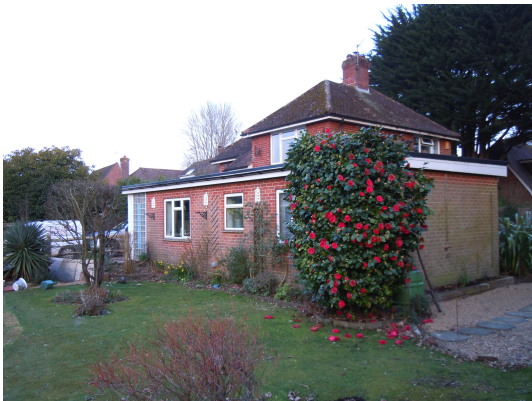
West and south west elevations
