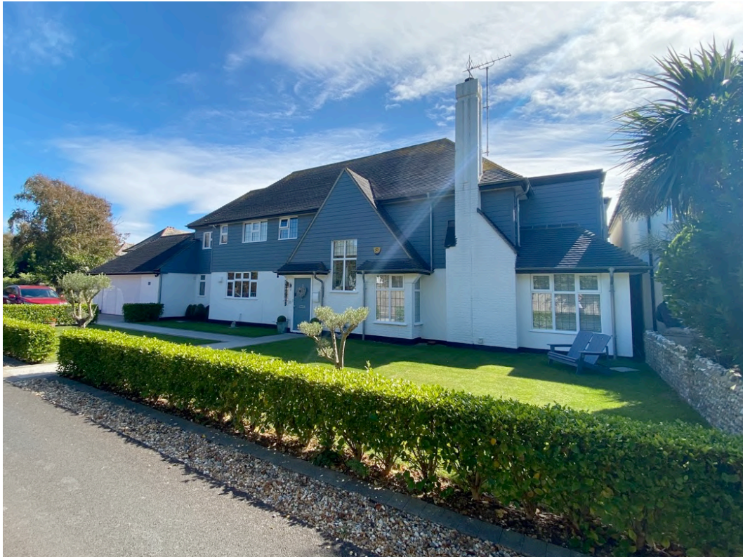
Front Elevation of 2 The Byeway
