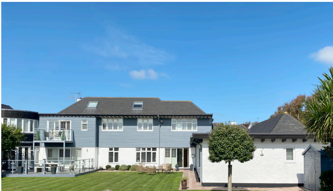
Rear Elevation of 2 The Byeway
