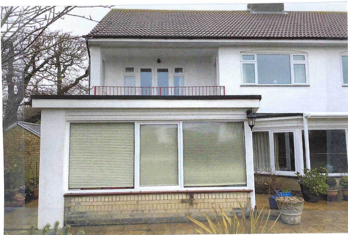
REAR PROPERTY SUN ROOM TO BE PART DEMOLISHED
