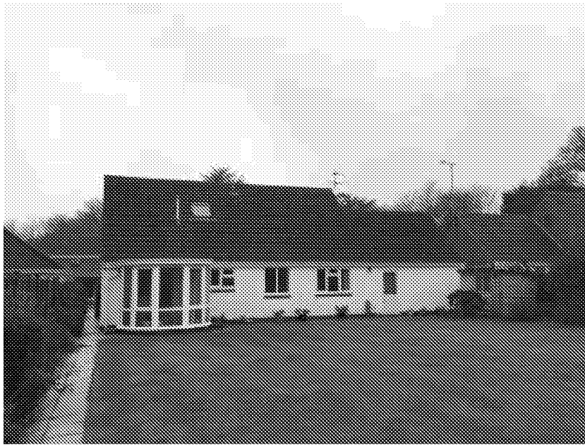
Photograph 01 – Existing North East elevation
