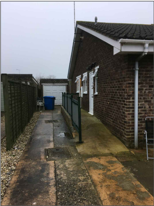
Existing Ramp Image
