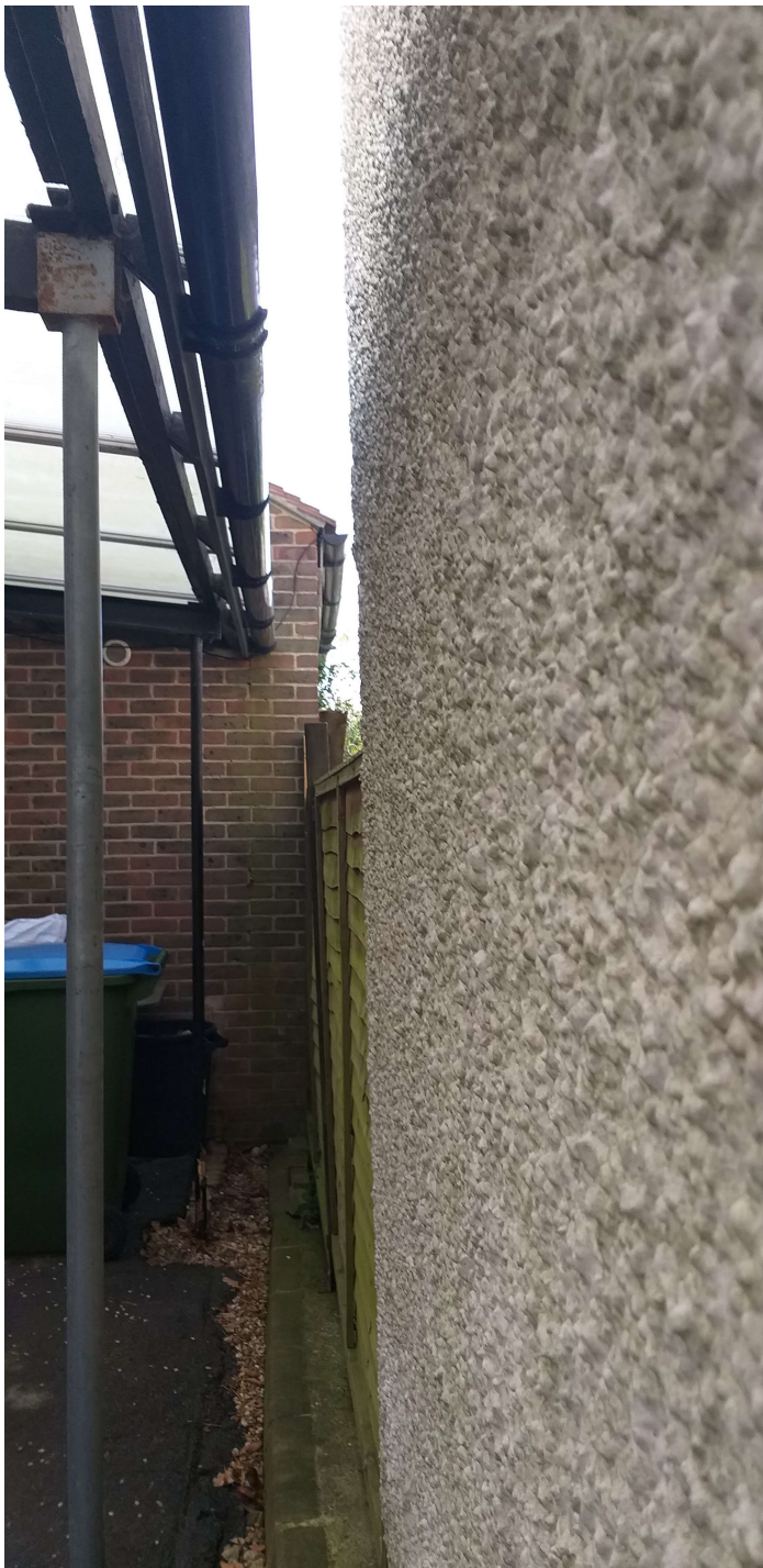
Existing carport front pier clear of adjacent wall tile canopy to be removed
