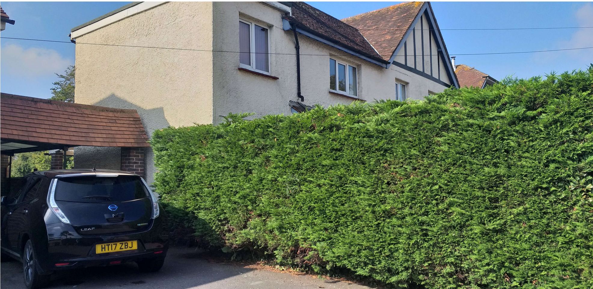
North West aspect existing front.
