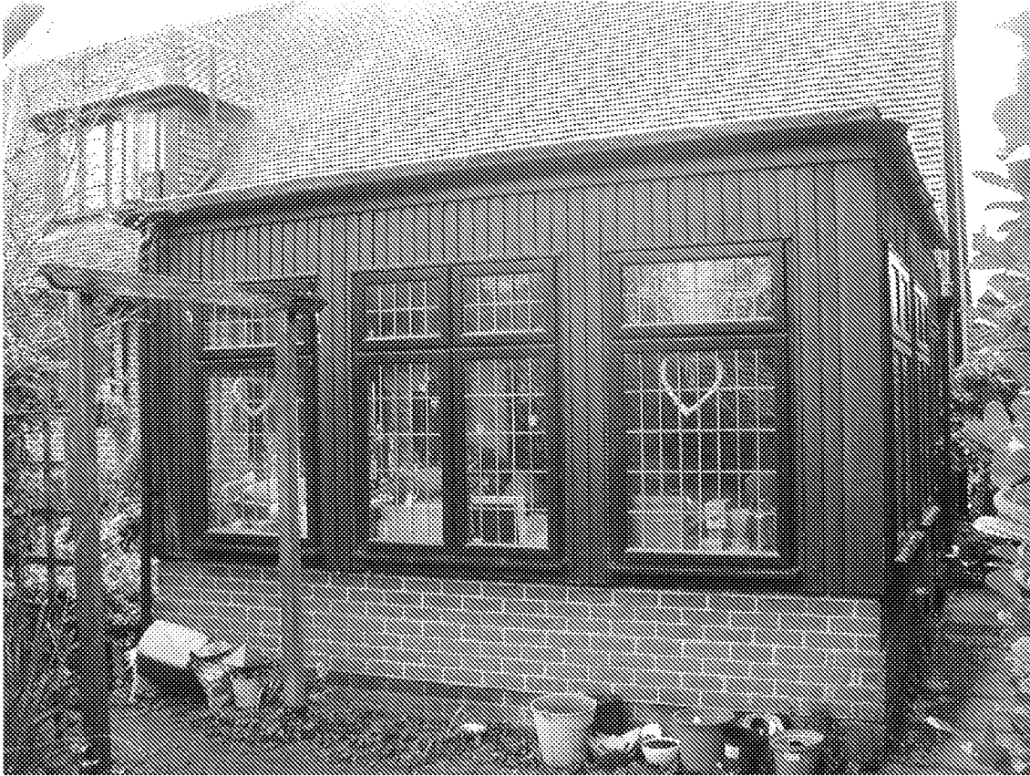
Picture – The existing sun room to the rear to be adapted and incorporated into the new development.
