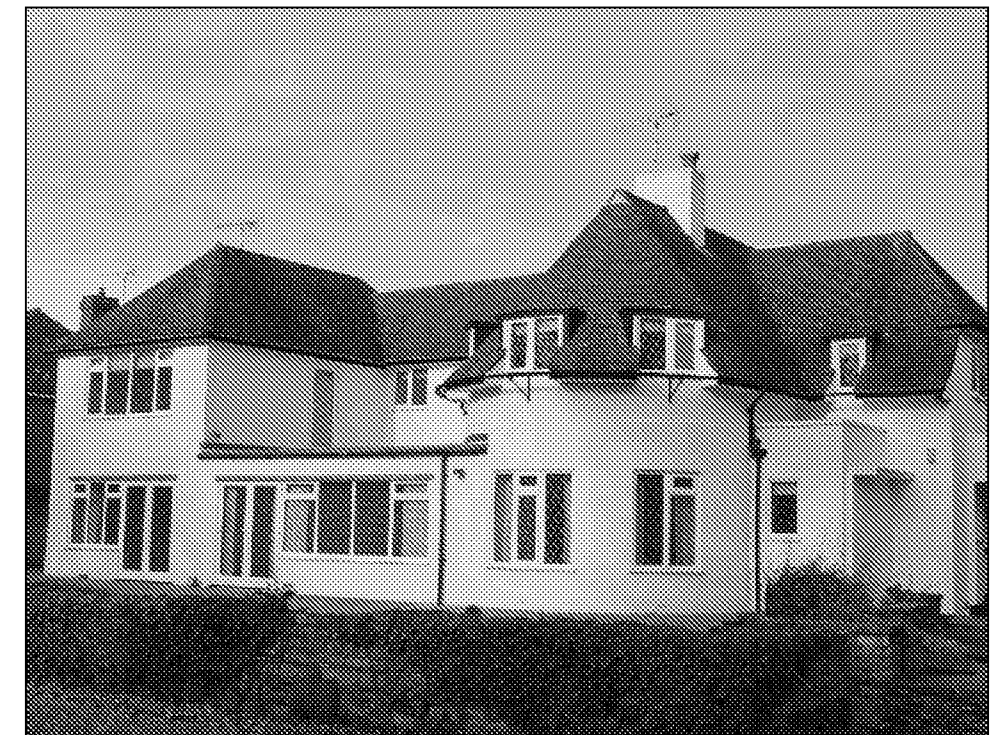
Existing property viewed from the southeast
