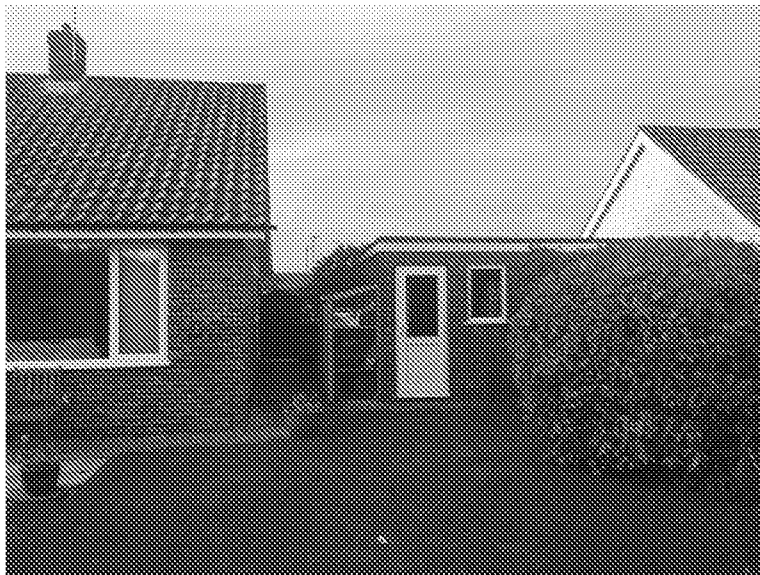
Part rear elevation of no. 15 with garage.
