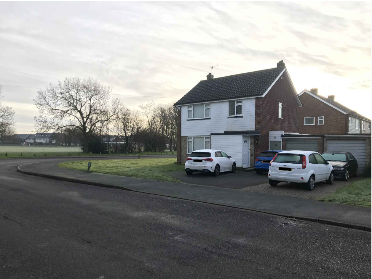
01 NORTH WEST CORNER
