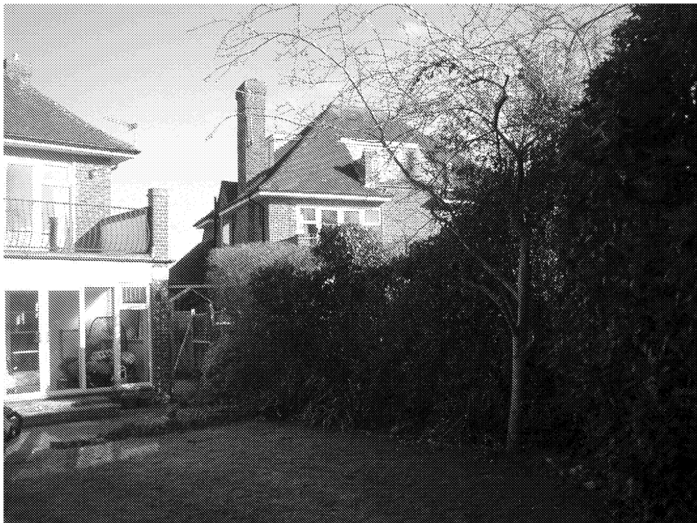
Pic – View of the other side of the house at the rear showing the Cherry tree and hedging.
