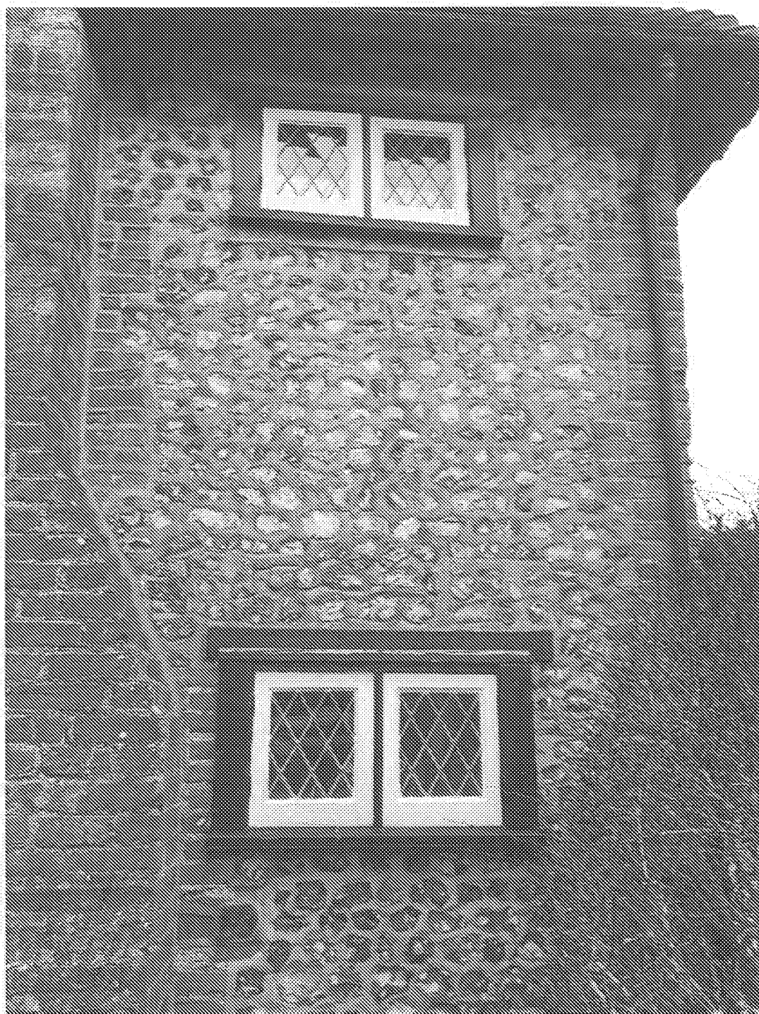
EXISTING WINDOWS TO RIGHT OF CHIMNEY – DOUBLE CASEMENT
