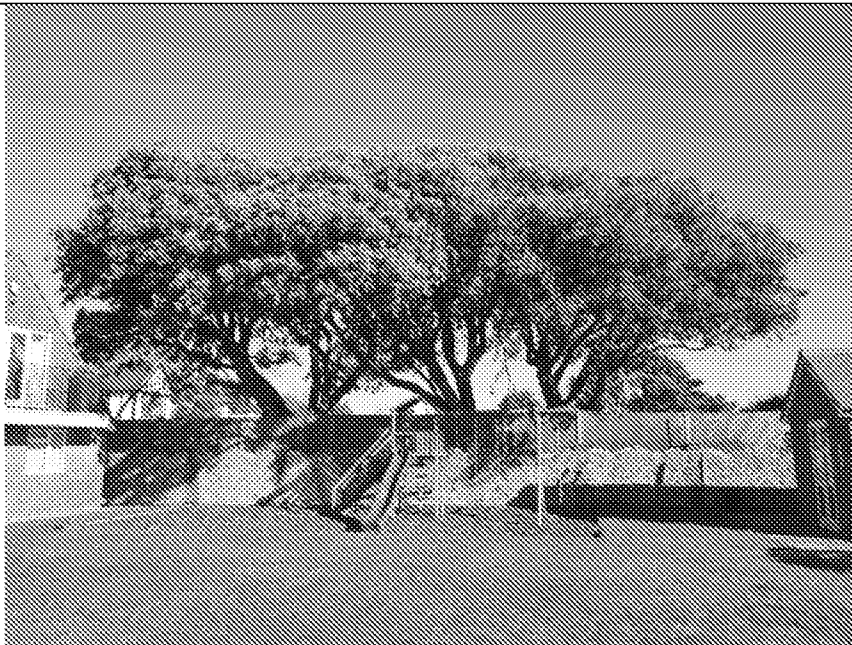
Picture 2. Overview of tree looking east from Sea Crest. Tree located atop of raised bank supported by a retaining wall
