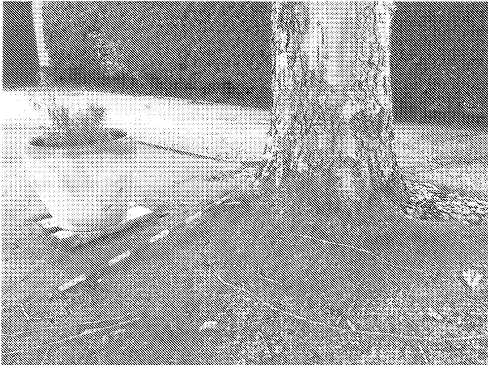
Showing proximity to the manhole and the main drain into the Aldwick Road
