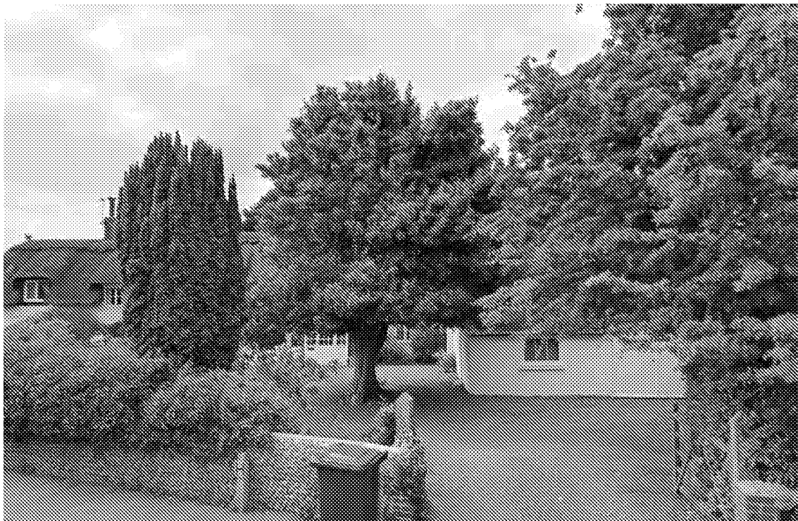
Fig 2: The listed building consists of two semi-detached cottages, with the larger of these being Bramble Cottage. The existing access to the dwelling from Rose Green Road would remain unchanged.
