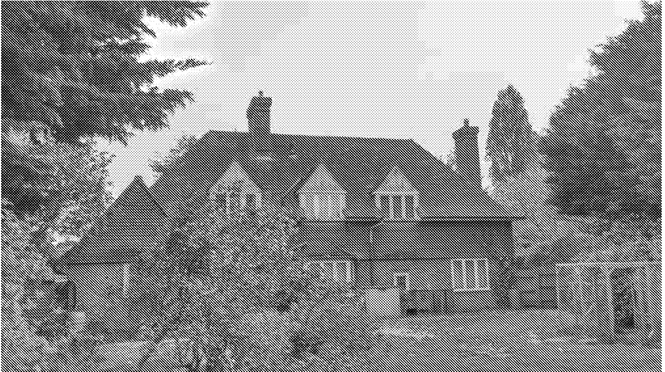
Photograph No. 1 - View of the dwelling to which the garden belongs. No detailed assessment of the dwelling has been undertaken as the dwelling is to be retained; however, the building is considered to offer suitability for bats.
